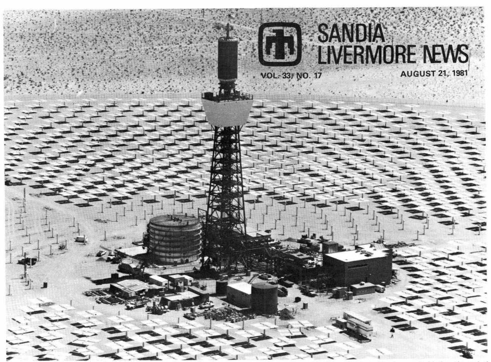
WORK IS PROGRESSING at the Solar One 10-megawatt electric pilot plant near Barstow, Calif., with more than 1100 of the 1818 heliostats installed by early July when this photo was taken. The thermal storage tank is completed and filled with the oil and rock and the 300-foot-high tower and solar central
